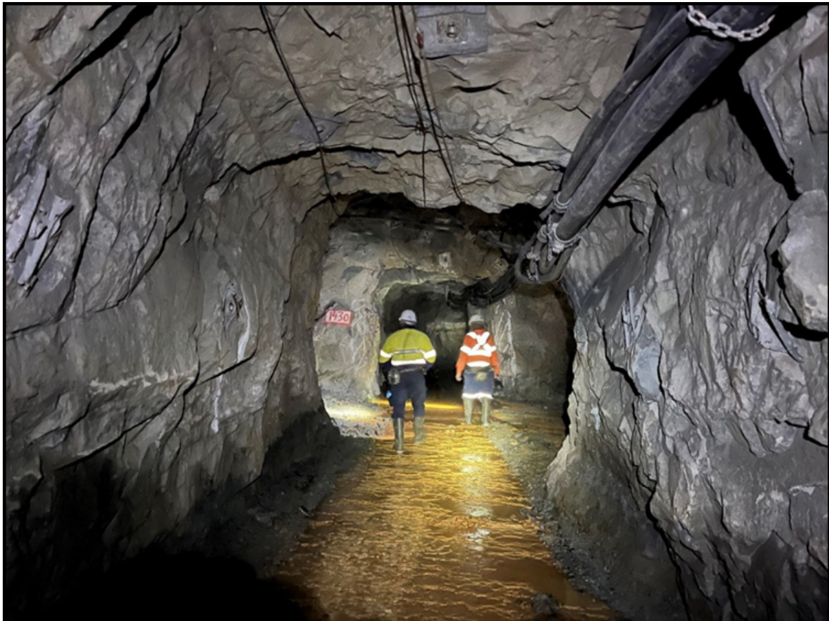
Figure 1 Looking along the Amalgamated Adit.
